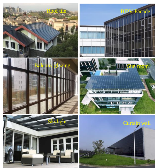
Fig.2 BIPV systems in actual construction scenarios [13].
